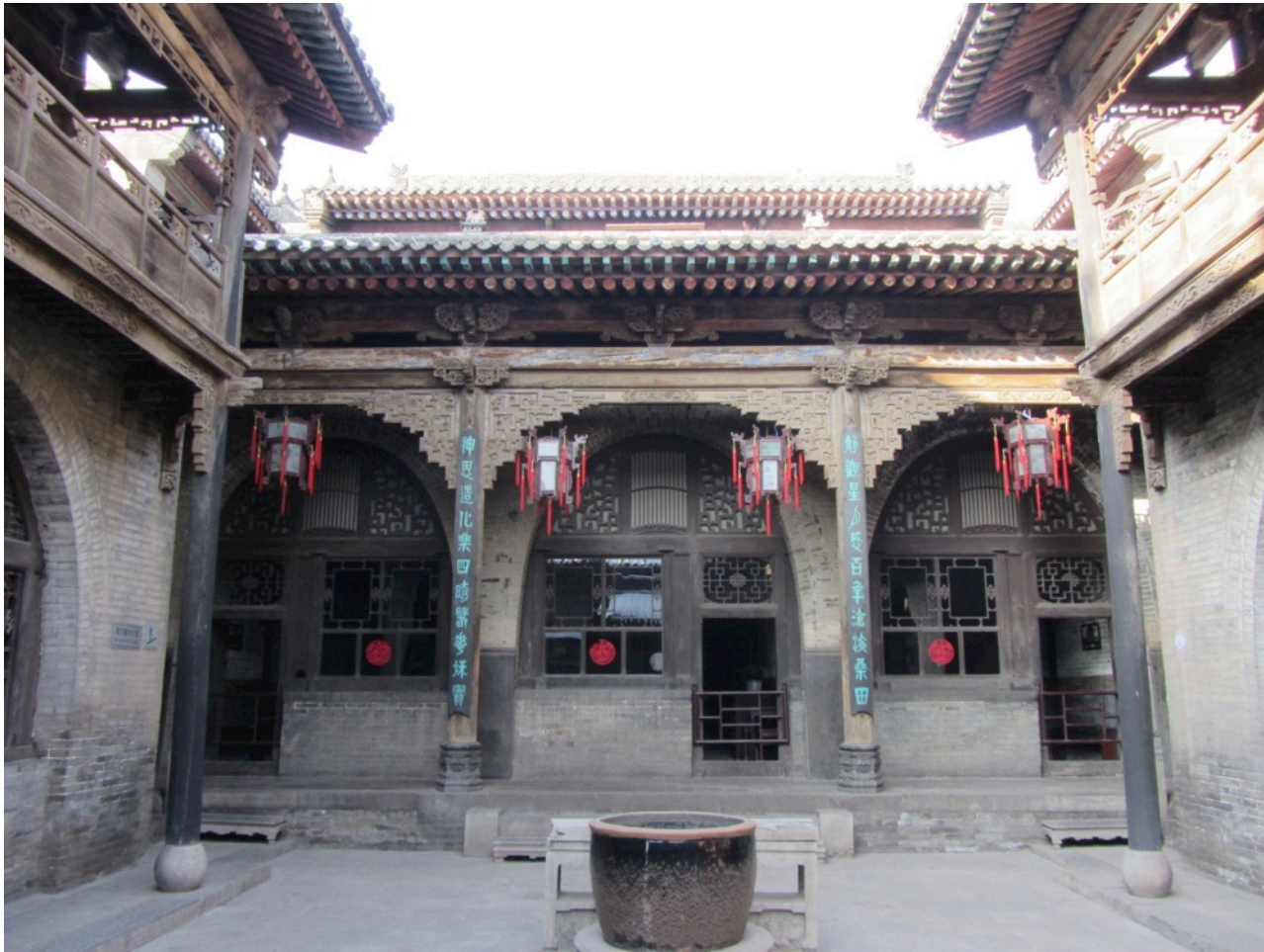
The middle courtyard
